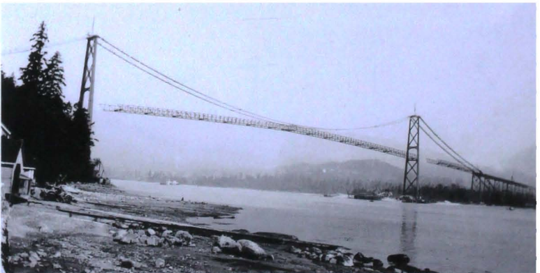
Lions Gate bridge construction, 1938
