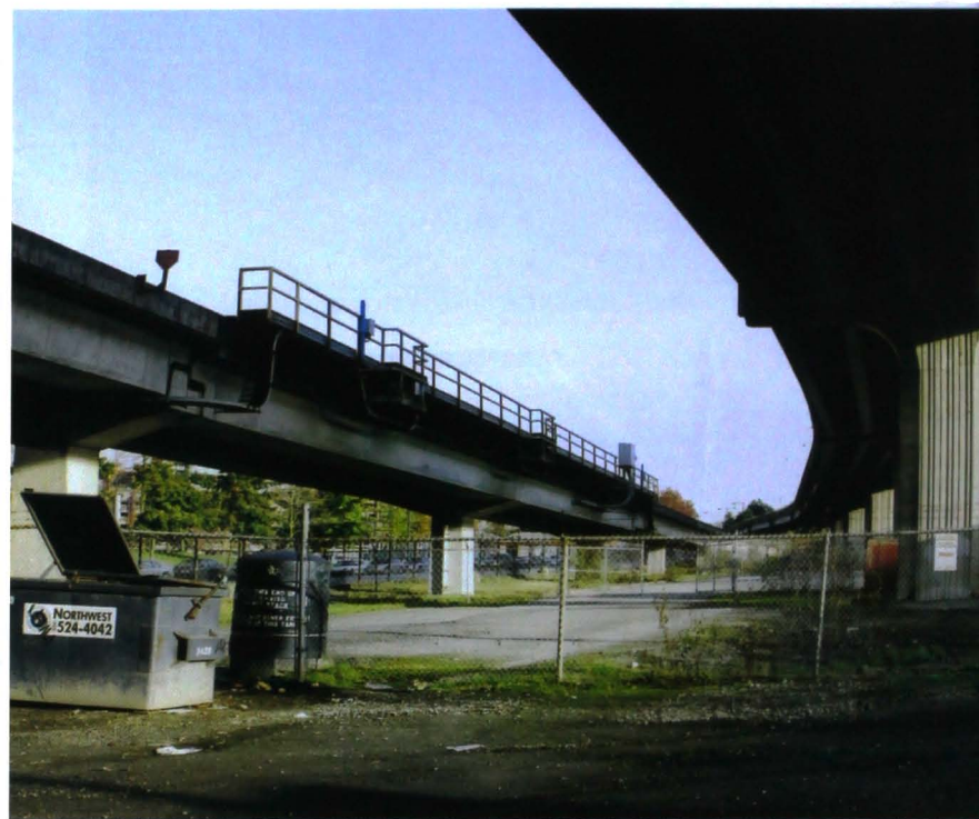
Georgia Street viaduct and Skytrain line
