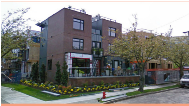
D) RS-1 ...emphasis is placed on the external design of all new buildings and additions being compatible with the historical CHARACTER of the area
