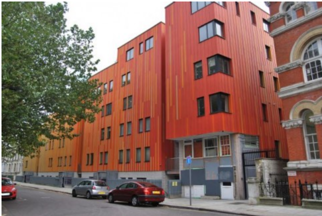
One interpretation of neighbourhood character. Wansey Street Housing, London. DRMM Architect
